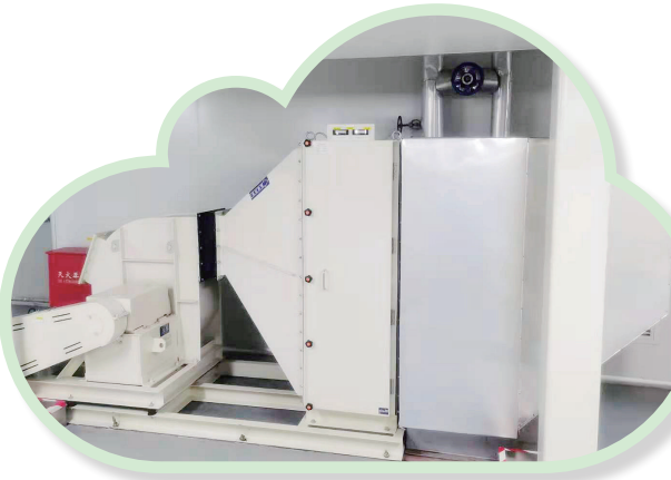
紫江新材料通过开展导热油锅炉排烟口热能回用项目改造，每年可节约天然气约 25,000 立方米，节能率约为 11.6%。 Zijiang Mew Material reuses the thermal energy at the smoke outlet of the heat-conducting oil boiler, which can save about 25,000 m³ of natural gas every year with an energy saving rate of about 11.6%.
